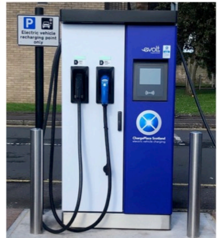
Journey (rapid) charger (50 kW DC, 43 kW AC)
