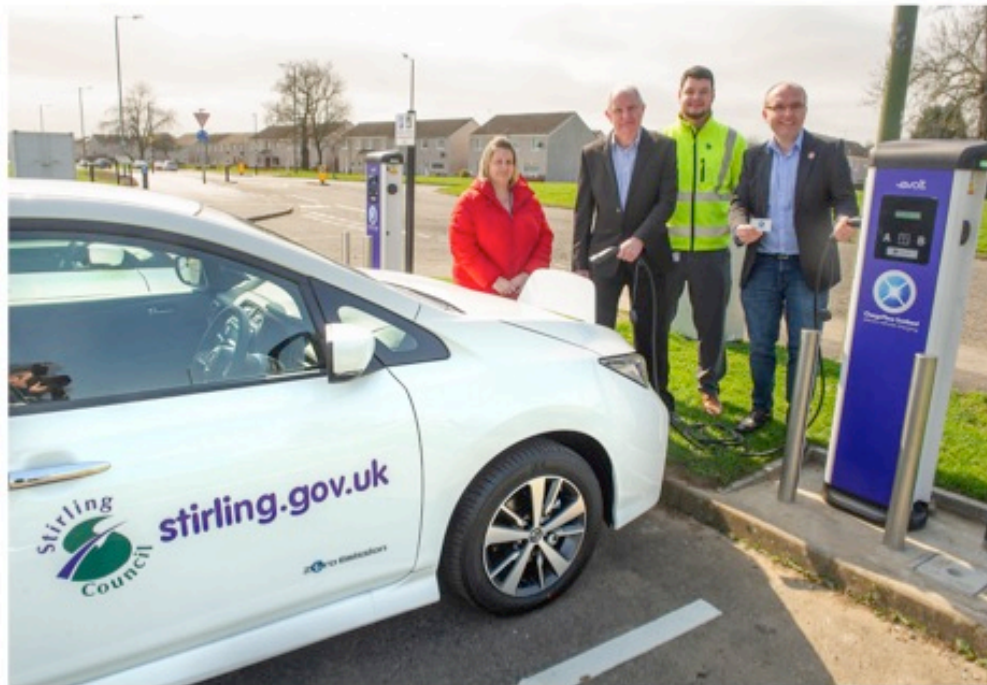
Destination (slow/fast) charger (7 kW / 22 kW AC) Other charging networks are available e.g Tesla, InstaVolt etc
